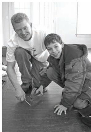
President David Baker and son, Kris, repairing the cottage
